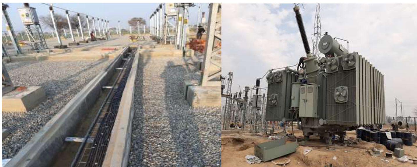
LAYING AND TERMINATE THE CONTROL CABLES
