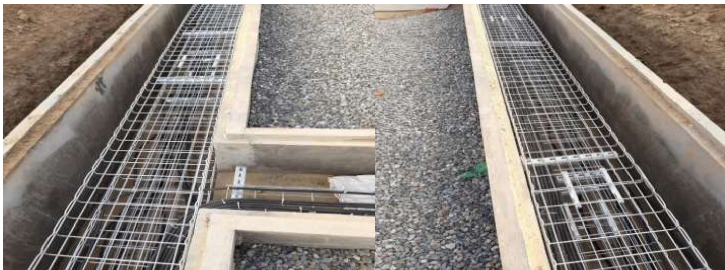
CABLE TRAY WORK AT 220/25 KV TRACTION SUBSTATION FOR RAILWAY
